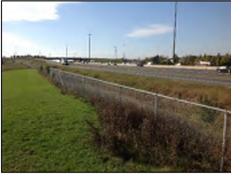
Image 11: Highway 400 and Rutherford Road Overpass facing southwest
