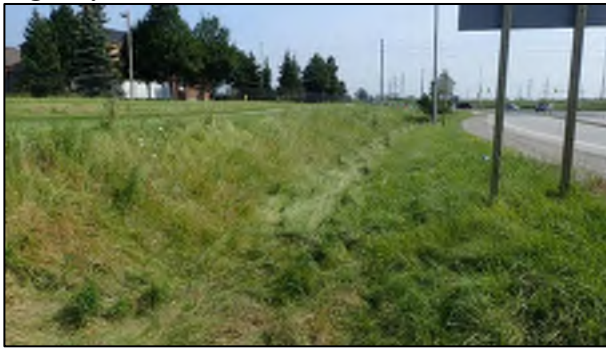
Image 91: Langstaff Road southeast towards Highway 7, note ditch
