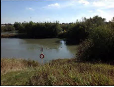
Image 9: SWM pond facing south
