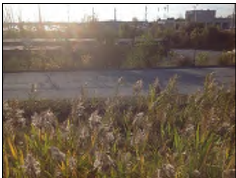
Image 53: Train tracks and internal road facing west
